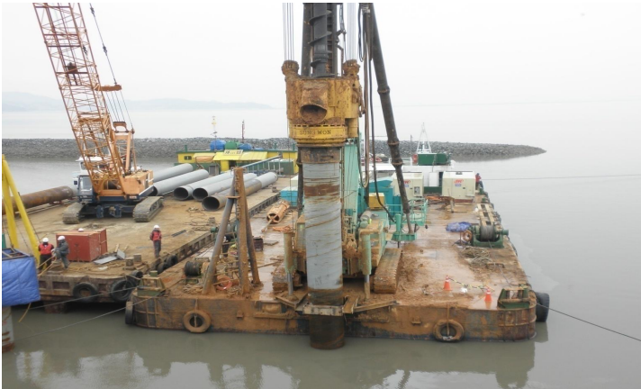
[ Percussing Rotary Drill : PRD공법 ]
